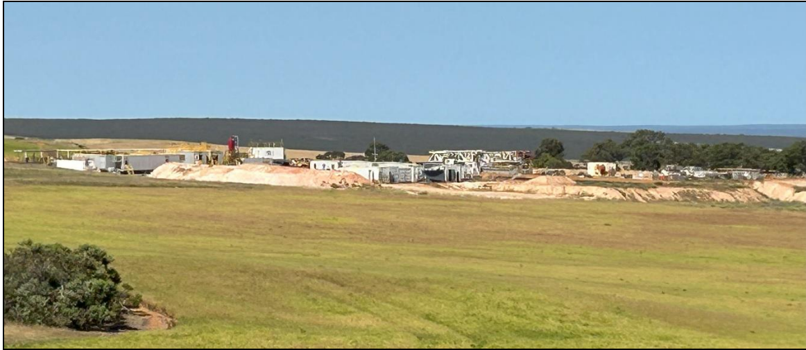
Figure 10.3.5 – existing drill site upon Lot 10710 Tomkins Road, Arrowsmith East
