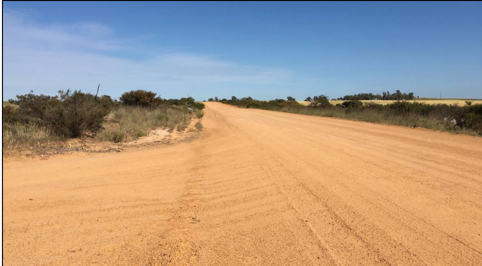
Figure 10.4.10 – View facing west along Skipper Road from eastern access point
