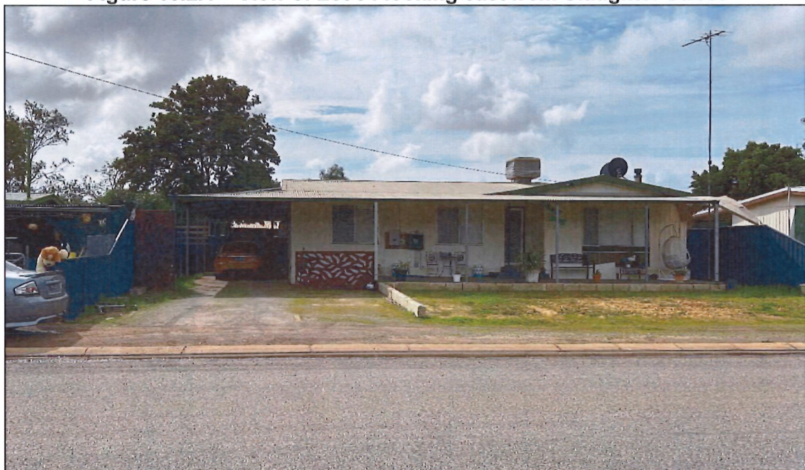
Figure 10.2.5 – View of Lot 34 looking north-west from rear lane
